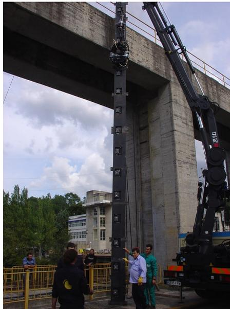
**Figure 5: A fully instrumented frame being moved into the intake bay at Velle**
