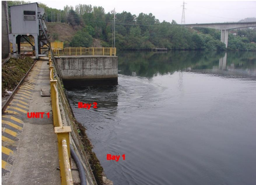
**Figure 12: The flow entering at a sharp angle in Bay 2 in Unit 1 at the Velle plant**
