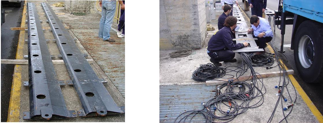
**Figure 4: ASFM frames (left) and ASFM components being installed (right - frame upside down)**
