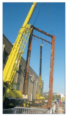
A view of the 30-path ASFM frame being lifted into the slot.
