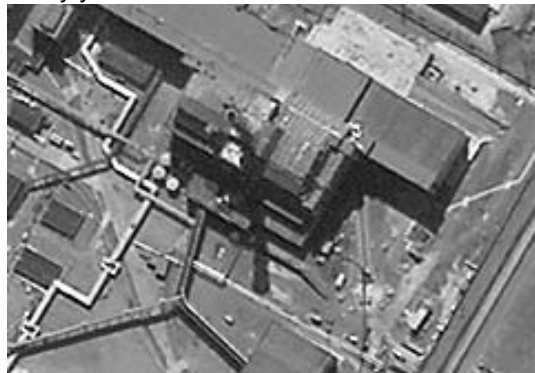
Figure 1. A high resolution EOS satellite image of the sarcophagus encasing the damaged nuclear reactor at Chernobyl, Ukraine [1].
